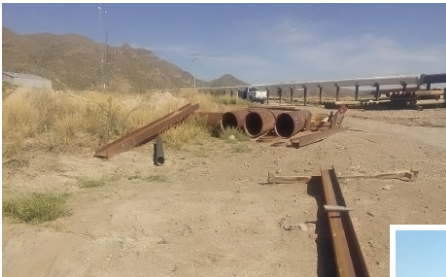
Work yard before
