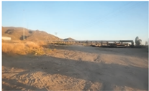
Work yard after
